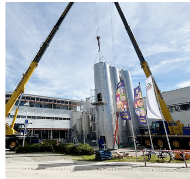
The brine tank farm was expanded as part of the capacity expansion in Schongau.
