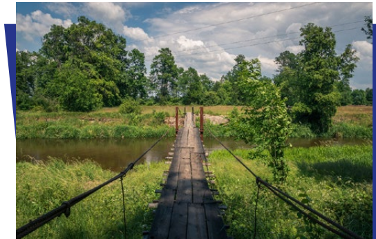
Photo: Footbridge across the Liwiec River
