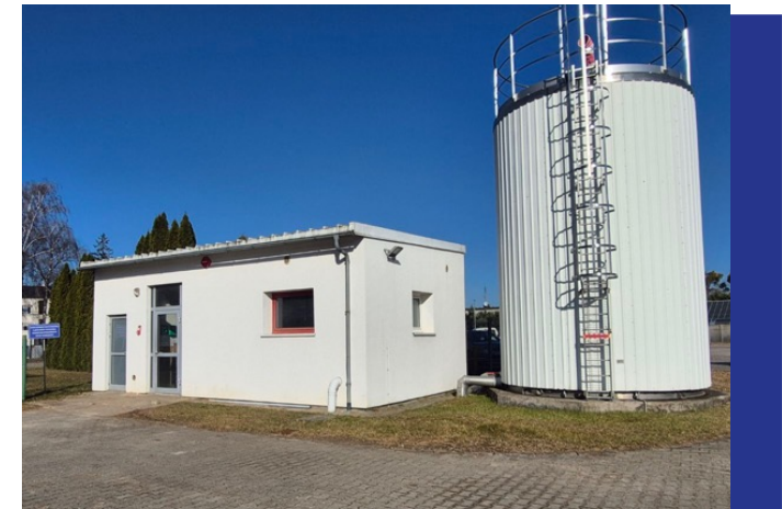
Photo: Water treatment plant and deep well
